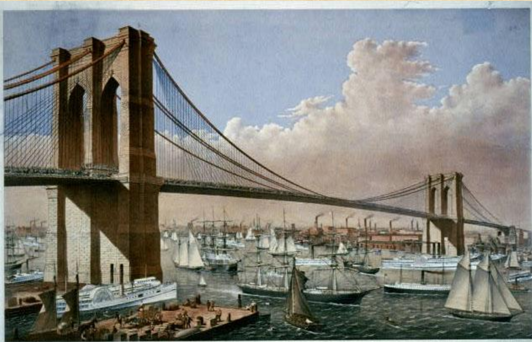
THE GREAT EAST RIVER SUSPENSION BRIDGE.
